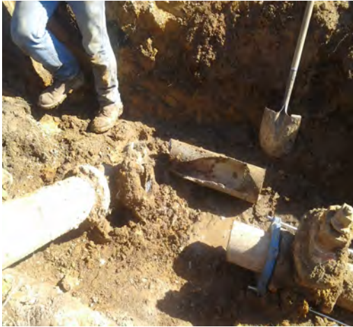
Contractors replacing water line
